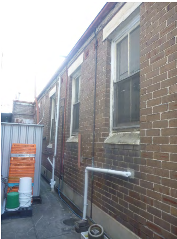
Figure 3.19 Eastern elevation of residence. (Source: GML August 2013)
