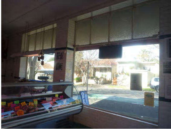
Figure 3.7 Internal view of the shopfront windows (facing south to Allen Street). (Source: GML August 2013)
