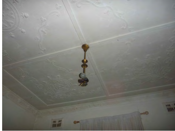
Figure 3.12 Decorative plaster ceiling and cornices in the residence living room. (Source: GML August 2013)
