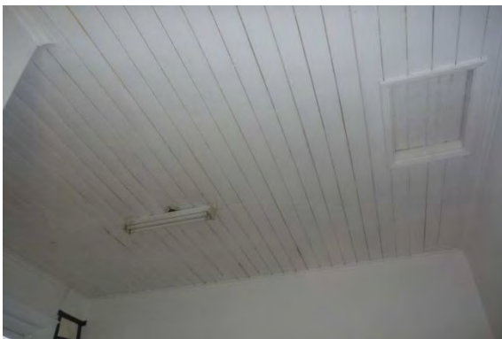
Figure 3.15 Timber ceiling in rear wing with simple timber board ceiling. (Source: GML August 2013)
