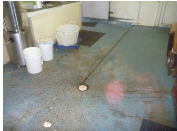
Figure 3.10 Concrete floor with falls to one drainage outlet in the 'boning room'. (Source: GML August 2013)
