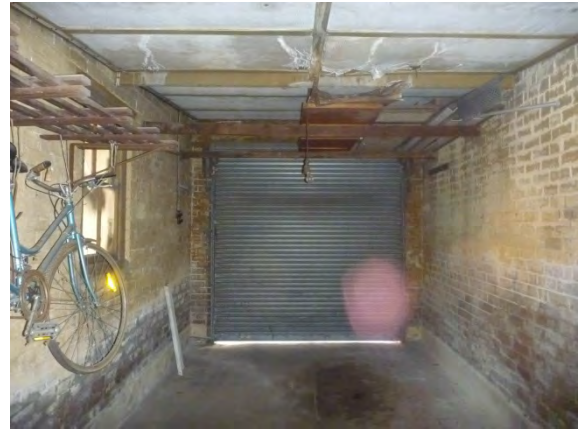
Figure 3.18 Internal view of the garage (facing west). (Source: GML August 2013)
