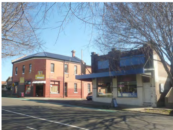
Figure 3.1 Allen Street relationship with No. 81 Allen Street opposite the subject building. (Source: GML August 2013)
