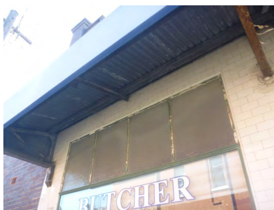
Figure 3.4 Original awning and window opening. However, window may have been replaced. (Source: GML August 2013)
