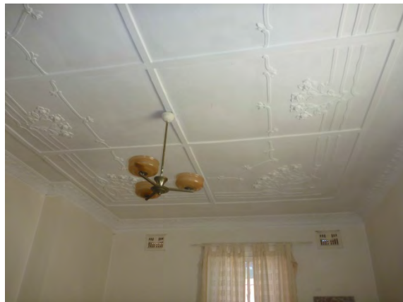
Figure 3.14 Decorative plaster ceiling and cornices in a bedroom. (Source: GML August 2013)
