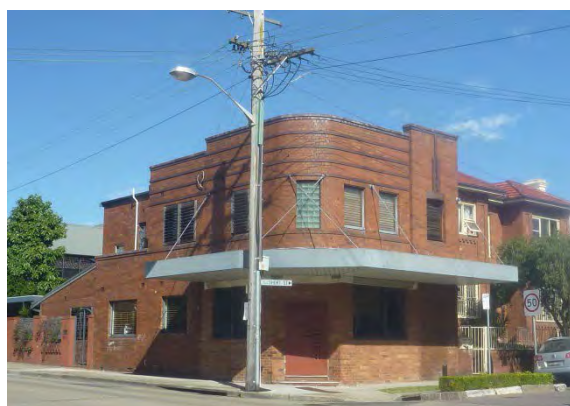
Figure 3.21 2 Short Street (cnr Balmain Road). (Source: GML August 2013)
