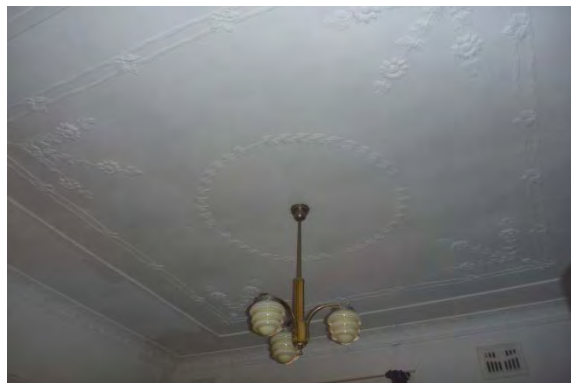
Figure 3.16 Decorative plaster ceiling and cornices in a bedroom. (Source: GML August 2013)
