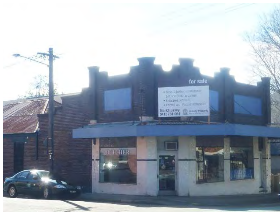
Figure 3.2 Primary frontage of the subject building at the corner of Allen and North Streets. (Source: GML August 2013)
