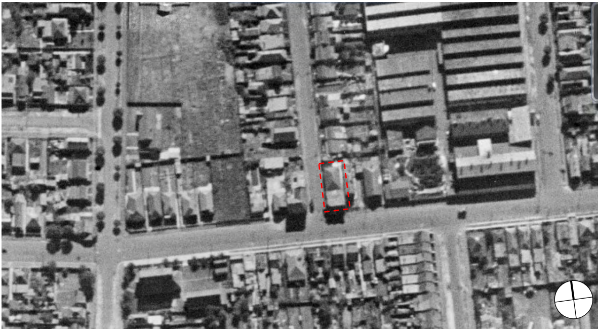
Figure 2.6 1943 aerial photograph of the site showing the Phase 2 Occupation buildings in the subject site (outlined in red) (Source: LTO)
